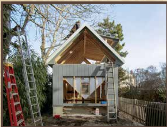
Hinge Roof Under Construction
