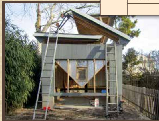
Jacking up Roof
