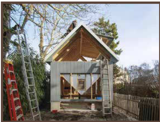
Hinge Roof Under Construction
