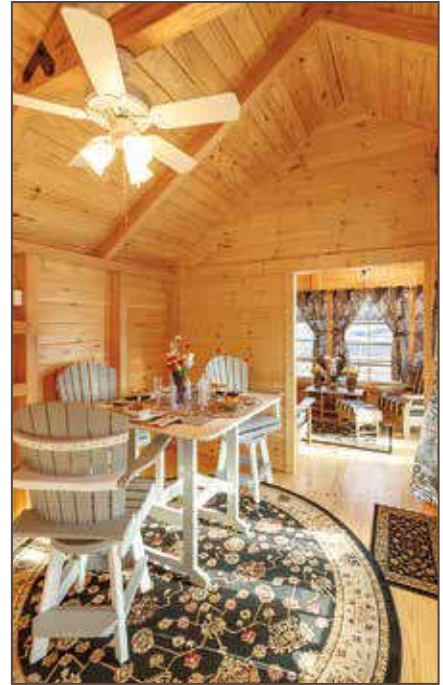
Timber Framing, Tongue and Groove Walls and Roof
