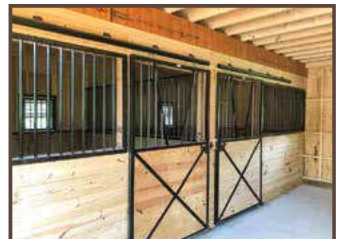
On-Site Build Horse Barn
