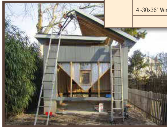
Jacking up Roof
