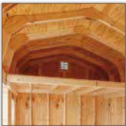
4' Deep Loft in Dutch Barn
