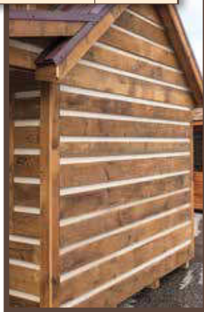
Old Reclaimed Siding with Chinking
