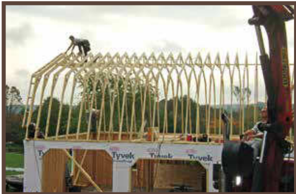
Build On Site
