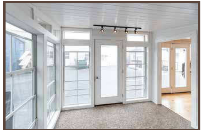
Azek Tongue and Groove Interior, Track Lighting and Carpet
