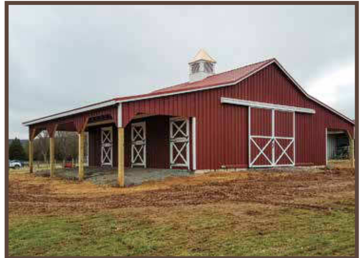
(523) On-Site Build Horse Barn
